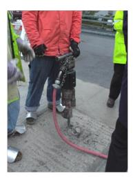
equipment. For example, jackhammers must be outfitted with noise-reducing mufflers and/or have portable street barriers to reduce the sound impact on the area. The Noise Code also defines the hours when construction may occur.
